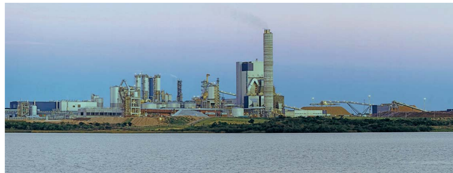
Andritz also delivered UPM's first pulp mill in Uruguay, which was started up in 2007 in Fray Bentos
