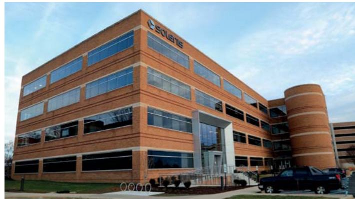
Solenis has moved to a new 90,000sqft global headquarters at Wilmington in Delaware
