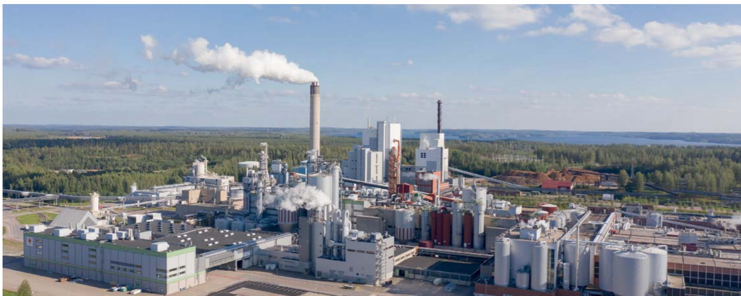
Stora Enso Imatra and ANDRITZ together developed how to locate the Flash Drying plant in an efficient space in the mill. The new Flash Drying Line was fitted into the overall layout
