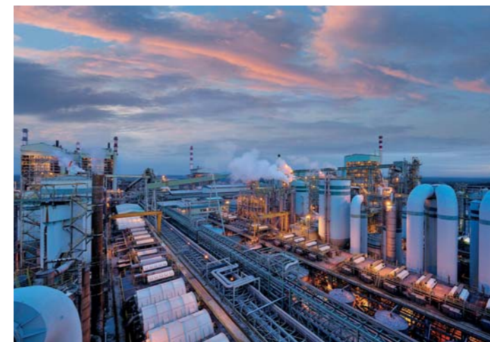
The Riau Andalan Pulp & Paper mill at Kerinci where chloride removal systems are being updated
