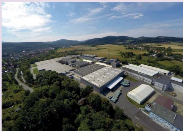
WEPA's mill at Piechowice in Poland where a tissue line is being installed by Toscotec
