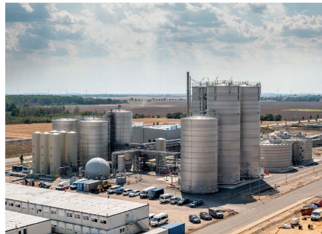
Closed water loop: All water used in production at Progroup AG's Sandersdorf-Brehna mill is cleaned in the company's own water treatment plant and then returned to the production process
