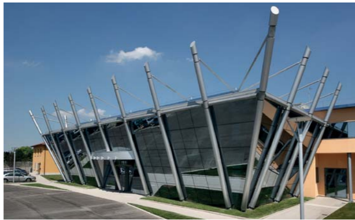
Fabio Perini's stylish facility in Bologna, Italy
